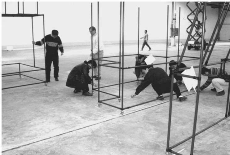
FIGURE 52.11 Construction of a physical mock-up for the gear machining cell charted in Fig. 52.9. (From Planning Manufacturing Cells © Copyright 2002 Richard Muther & Associates.)
